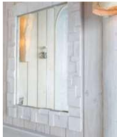
2.1.5 Wooden blocks re-used for wall panelling
